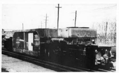
FIRST G-E DIESEL-ELECTRIC LOCOMOTIVE BUILT FOR UNDERGROUND MINING SERVICE.
