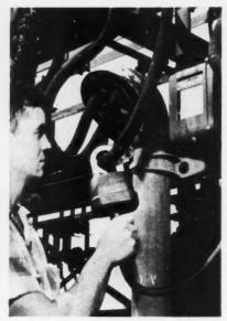
**SYSTEM SURVEYS** up to 8.7 kv are now practical with butyl-molded hook-on transformer.
