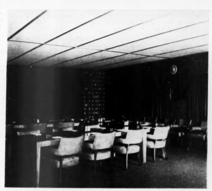
**LUMINOUS CEILING** that can be dimmed was installed at Ford Motor Company's conference room in Detroit, Mich. It has a range of illumination from one-half to 60 footcandles.
