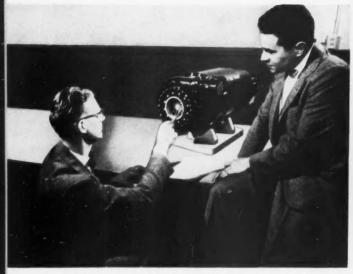
FIRST COMPLETELY SELF-CONTAINED air-turbine-driven hydraulic pump for an aircraft hydraulic system, and the first successful air-
