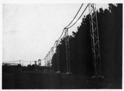
PREASSEMBLED AERIAL CABLE, insulated with varnished cambric, was installed at the Highland Cotton Mills, High Point, NC. Parallel feeders carry power to five load centers.
