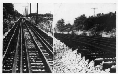
TEST TRACKS PERMIT STUDY OF LOCOMOTIVE REACTION TO ABNORMAL TRACK CONDITIONS.
