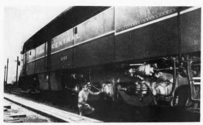
NEW EQUIPMENT DETECTS, INDICATES, AND CORRECTS WHEEL SLIP IN THREE SECONDS.
