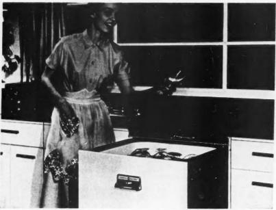
UNDERCOUNTER DISHWASHER CAN BE LOADED WITHOUT REMOVING OR SLIDING THE RACK.
