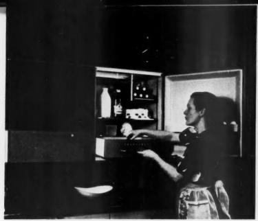
**REFRIGERATOR-FREEZER** of the future has one-half-inch-thick walls, magnetically sealed doors that open from kitchen and dining areas, and an ice-water tap.
