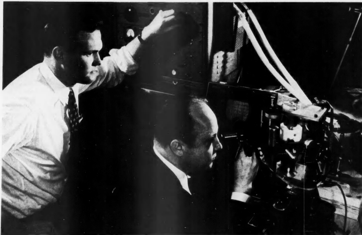
RESEARCHERS CROWE (LEFT) AND SHARBAUGH STUDY THE CHARACTERISTICS OF AN INSULATING OIL UNDER HIGH-VOLTAGE STRESS.
