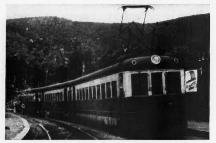
LOCAL PASSENGER SERVICE on electrified railroads in the countries of Brazil and Chile is often handled by multiple-unit trains made up of one motor car and two trail cars.
