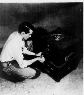
PRESSURE-RELIEF VALVES ARE PROTECTED BY COVER ON CONTAINER FRONT. BOLTING COMPLETES JOB. NEW WAY IS 80 PERCENT TIMESAVER.
