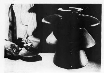
**OLD AND NEW:** Modern radio-noise-free pin-type insulator of porcelain for high-voltage transmission lines over-hadows 1906 design --still usable after 17 years of service.
