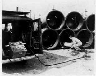
LEVEL-CHECKING X-RAY UNIT IS EFFICIENT AT HIGH PRODUCTION SPEEDS; PORTABLE INDUSTRIAL X-RAY UNIT MAKES A 360-DEGREE SWEEP.
