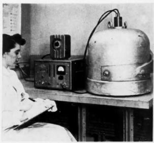
GAMMA RADIATION checked with scintillation counter indicates the abrasiveness of a plastics molding compound on metal-mold parts.
