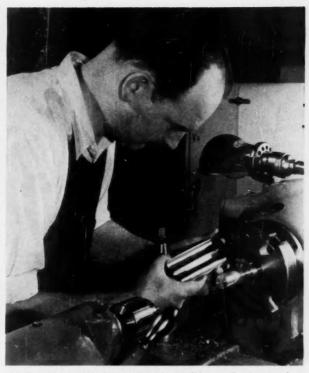
CYLINDRICAL-ROUGHNESS SCALES simplify specification, production, and inspection of the roughness of curved machined surfaces.
