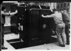
COOLING TUBES of vault-type network transformers are arranged in new design.
