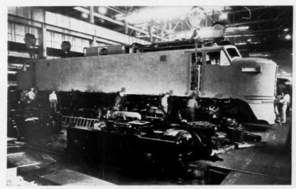
RECTIFIER-TYPE ELECTRIC LOCOMOTIVE WILL HAUL 18-CAR TRAIN ON THE NEW HAVEN.
