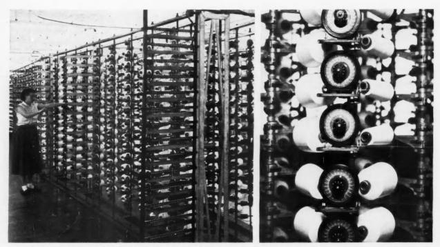
YARN-TENSION BRAKE USED ON WARPING CREELS IN TEXTILE INDUSTRY IS BUT ONE OF MANY APPLICATIONS FOR HYSTERESIS DEVICES.
