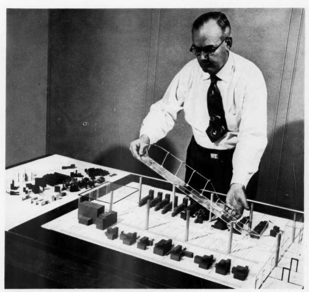
AUTHOR CARTER ATTACHES OVERHEAD PLASTIC CONVEYOR ASSEMBLY TO BUILDING STRUCTURE OF A THREE-DIMENSIONAL MODEL LAYOUT.
