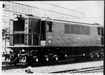
**DIESEL-ELECTRICS** having a G-E box cab invaded the passenger field in the mid-30's with 12 times the power of the early "oil-electric."
