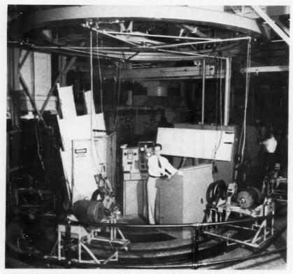
**MERRY-GO-ROUND** testing apparatus gives motors a final and different operational check at each station. The operator initiates tests from control consoles at center.
