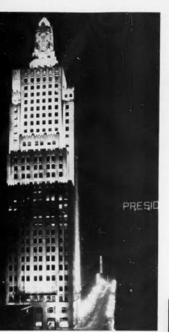
ACCENTUATING HEIGHT of Kansas City Power and Light Co. building in Missouri, illumination gradually tapers off at upper surface of each level. Suburban buildings (right) are easiest to illuminate because floodlights can be mounted at ground level and concealed by shrubbery.
