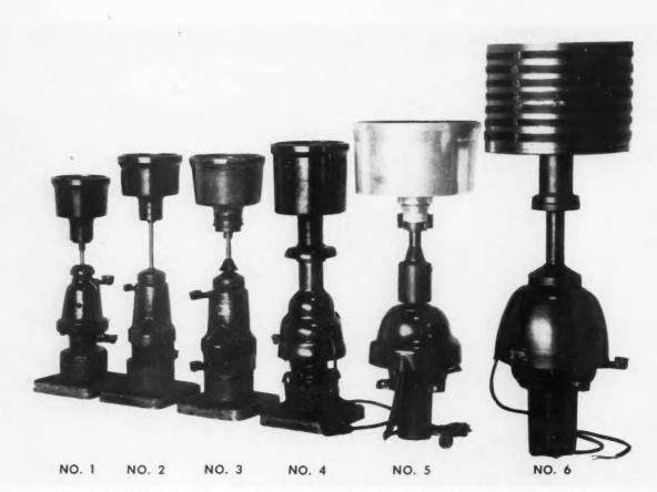
FROM THE FIRST ELECTRIC SPINDLES, MOTORS DELIVERING 3 HP HAVE EVOLVED TO DRIVE 16-INCH BUCKETS AT SPEEDS OF 10,000 RPM.
