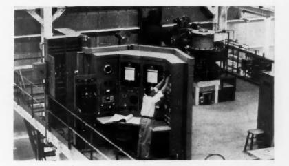
**SINGLE OPERATOR** at control console remotely operates the consummable-electrode arc-melting furnace in background. He views the entire melting operation by means of a closed-circuit system of television.
