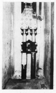
Termination of 2500 MCM, 15 kv silicone-rubber-insulated cable in Con Edison's Hell Gate generating station, stress cone completed on cable at left, in process on cable at right.
