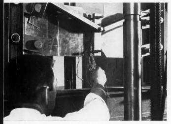
NOTCH TEST of metal plate is carried out in mechanical laboratory. Electric strain gages record the slightest bend.
