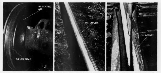
**OIL LEAKING FROM JOURNAL BOX** spreads over the wheel face (left) and onto the tread. When the oily tread strikes the rail, a
