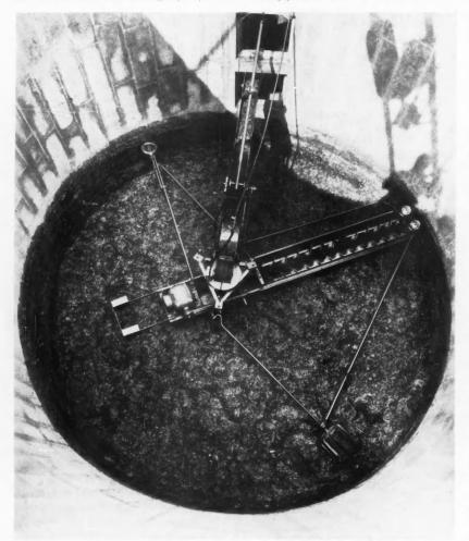
**INTERIOR SILAGE HANDLING:** Unloader throws silage through silo's portholes to feeding carts in the barn. On 75 New York farms, moving belts deliver silage directly to the cows.
