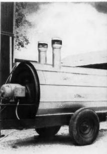
BALING Tractor-mounted generator, new concept of mobile power, not only permits electrifying trailing equipment but also furnishes emergency power.
