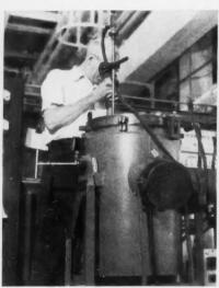
**NEW AND OLD**—Metallurgist shovels chemical into modern electric are furnace (left). Operator (above) measures temperature of melt inside 15-year-old vacuum furnace designed by laboratory scientists.
