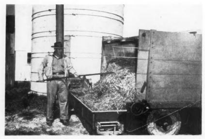
**EXTERIOR SILAGE HANDLING:** Electric-driven wagon unloader dumps grass silage into blower that sends it into storage by way of the vertical pipe outside of the silo.
