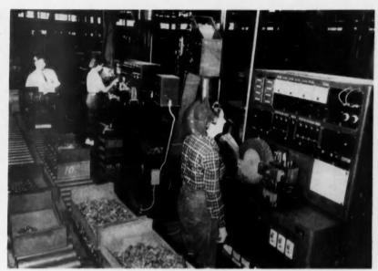
TWO AUTOMATIC MINIATURE PRODUCTION LINES INSPECT AND TEST LOUDSPEAKER MAGNETS.
