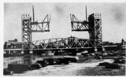
SELSYN CONTROL MAINTAINS LEVEL OF INDEPENDENTLY POWERED TWIN LIFT-BRIDGE SPANS.
