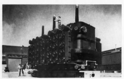
EXTRA COOLING CAN RAISE RECORD TRANSFORMER RATING OF 300,000 KVA TO 315,000-
