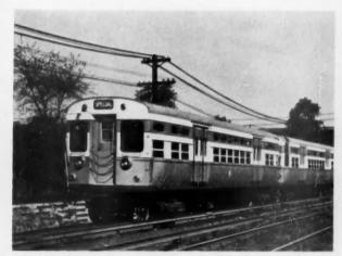
IMPROVED DESIGN of control and motors gave lightweight rapidtransit cars more horsepower per pound at little weight increase.
