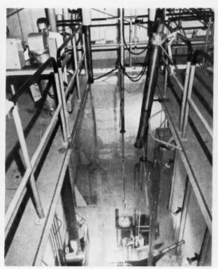
COLOR TV VIEWS WORKING ZONE IN CHEMICAL FACILITY. UNDERWATER TANK PERMITS SAFE EXAMINATION OF IRRADIATED FUEL ELEMENTS.
