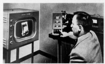
IMAGE OF INSPECTED PART APPEARS ON TV SCREEN FAR FROM SOURCE OF DANGEROUS X RAYS.
