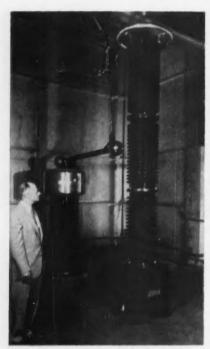
**COUPLING CAPACITORS** of high capacitance were put into production during the year.
