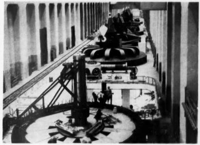
TWELVE 73,684-KVA HYDROGENERATORS FURNISH GENERATING CAPACITY FOR McNARY DAM.
