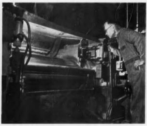
**DOUBLE-ROLL SYSTEM** rapidly turns out superior high-bulk-density molding materials with minimum of attention from an operator.
