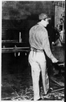
**4** Build-ups are stacked one on the other, with a separator sheet between, and heated in a large hydraulic press, one press handling many build-ups. When this curing process is complete, individual sheets of each build-up are fused into a solid laminate. **5** A separated four- by eight-foot Textolite laminate is now trimmed of all its rough edges on a giant shear cutter. Next, its smooth
