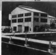
IN GAS PIPELINE PUMPING, G-E units lower pumping costs. G-E gas turbines are ideal for these installations as they go on the line in less than 15 minutes, can operate virtually unattended, use gas from pipeline as fuel. Little or no water, only a small amount of lubricating oil are required.
