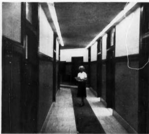
gives impression of greater width (left). Six-inch-wide recessed troffers equipped with rapid-start lamps and located at each side of the hall brighten walls and suggest space.
