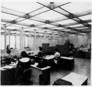
nous ceiling has environment-control features such as perforated wedges to regulate sound; some wedges introduce conditioned air. High-frequency high-voltage distribution system operates lighting.
