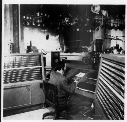
grams are viewed both in the studio and on monitors. The complex electronic control console (arrow, left and photo, above) operated by technicians manipulates each lamp individually.
