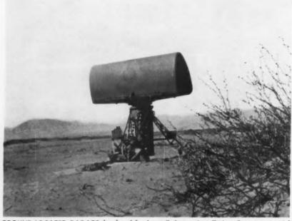
**GROUND-LOCATED RADARS** developed for Army Ordnance installations form an essential part of the beam-riding missile guidance system by directing the Nike to its target.
