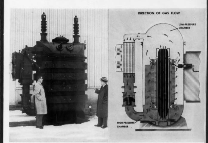
PROTOTYPE OF GAS-INSULATED SINGLE-PHASE 1000-KVA TRANSFORMER IS EXAMINED BY AUTHOR (RIGHT); GAS FLOWS IN ARROWED PATHS.
