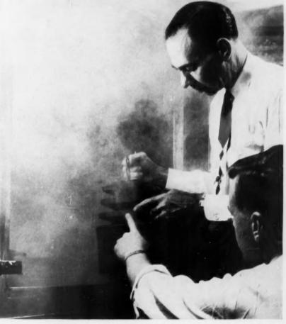
TRANSFORMER UNDERGOES EQUIVALENT OF YEARS OF EXPOSURE IN SALT-FOG CHAMBER.
