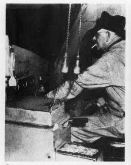
2 Hand on throttle, hostler prepares to move the million-dollar development locomotive out of the diesel shop to the ready track for its train.
