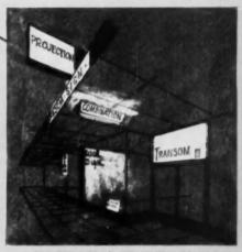
**MOUNTED IN A NUMBER OF WAYS,** luminous plastics signs identify individual stores grouped under protective canopy. Fluorescent lamps, satisfactorily operating down to zero F, provide even illumination. Various lettering styles and colors are used.
