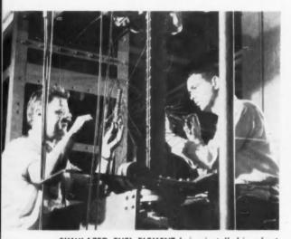
**SIMULATED FUEL ELEMENT** being installed in a heat transfer loop for tests under reactor thermal conditions. This is one of G.E.'s supporting atomic development programs to advance reactor design.
