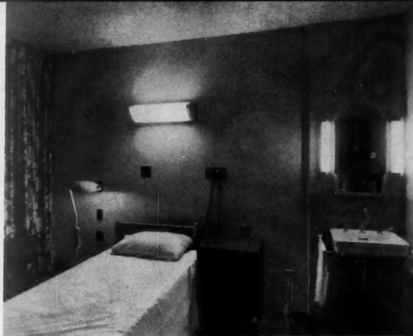
Patients' Rooms Forty-watt fluorescent lamps in wall bracket above beds provide pleasant general lighting (left). A luminous wall unit, suitable for private rooms, can be used for reading, night lighting, and examinations.
