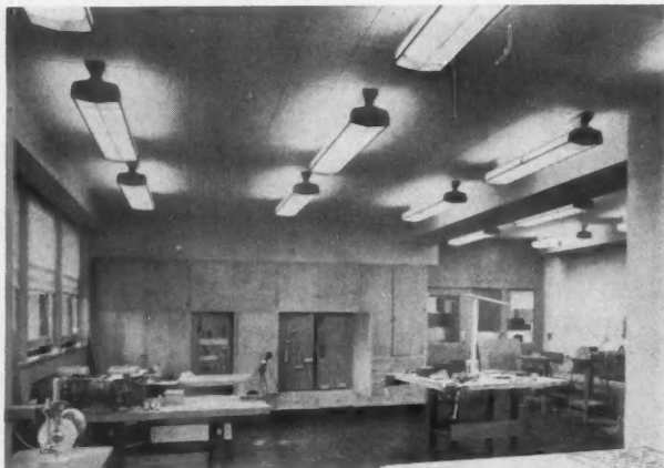
Occupational Therapy Good lighting lessens the strain and fatigue of the physically handicapped (left). Well-shielded commercial-type fixtures for shop training reduce glare and help prevent accidents.
