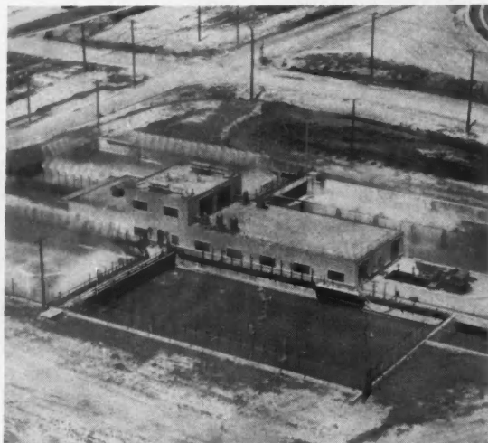
Cooling Ponds collect warm, used water and speed evaporation by the use of low-pressure sprays.
