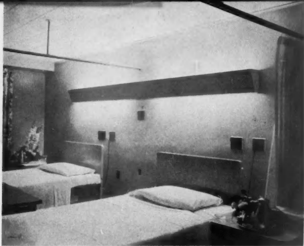
Patients' Rooms Forty-watt fluorescent lamps in wall bracket above beds provide pleasant general lighting (left). A luminous wall unit, suitable for private rooms, can be used for reading, night lighting, and examinations.
