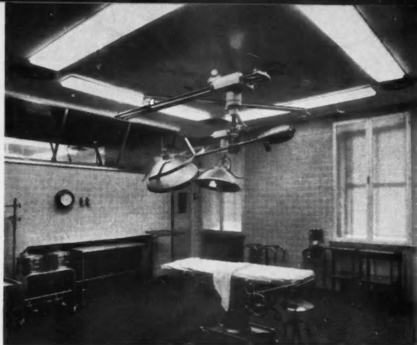
Surgery Fluorescent lighting plays an important role in operating areas. Built into ceilings, it supplies "fill-in" light in much the same way as on a regular theater stage—giving shadowless illumination for better working comfort.
