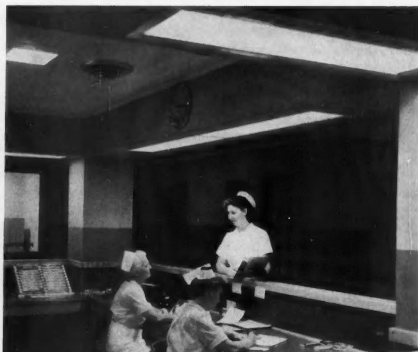
Corridors and Nurses' Stations Cove lighting on one wall spreads diffuse light, adding to apparent ceiling width (left). Well-shielded fixtures also give good diffuse lighting, reducing glare.
