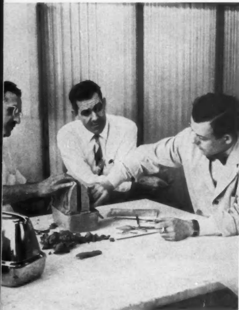
MODELMAKERS apply plasticene to clearance skeleton while Rawson (center) watches.
