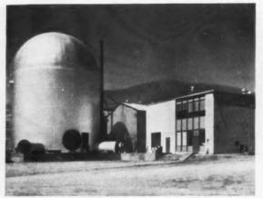
**PURPOSE OF EXPERIMENTS** to be conducted in Developmental Boiling Water Reactor is to develop economic nuclear power. Facility will furnish steam to 5000-kw turbine-generator, owned and operated by Pacific Gas & Electric Company.
