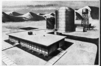
**GENERAL ELECTRIC TEST REACTOR**, planned for completion in 1958, is a new concept in reactor design developed by General Electric. This 30,000-kw test reactor combines features of tank and pool reactor types.
