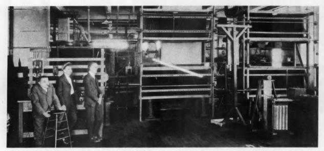
MAN-MADE LIGHTNING, a valuable contribution, enabled engineers to laboratory test resistance of electric equipment to lightning.
