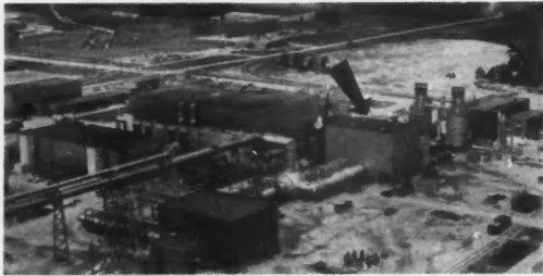
USAF's wind-tunnel center includes an engine-test facility (arrow), where air-breathing propulsion systems are tested inside sealed cells (right).
