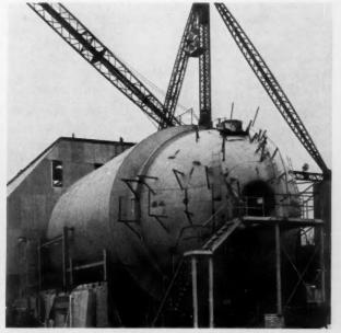
SUBMARINE HULL SECTION at the KAPL West Milton site will house the prototype atomic power plant for the submarine Triton.
