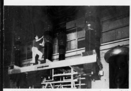
AIR-BLAST CIRCUIT BREAKERS improve interrupting efficiency and operating speed with newly designed interrupter elements mounted within their own high-pressure air-storage tank.
