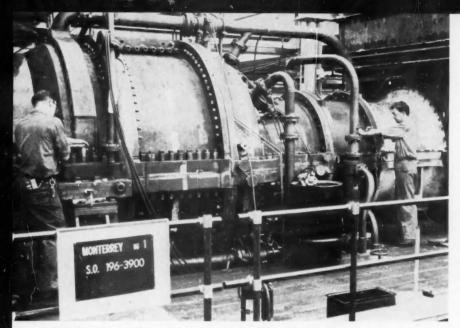
GAS TURBINE, rated 16,500 kw and one of the largest ever built, operates in Mexico.
