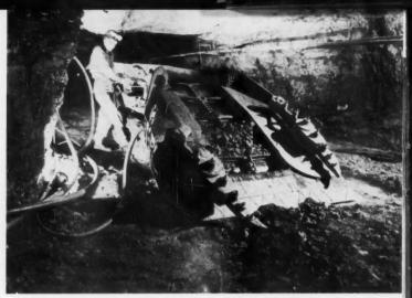
**PORTABLE CABLE** with Y-shaped ground conductor augments today's 3-phase a-c mining equipment, has long life in rugged service.
