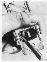
WIRING DEVICES in a line can be easily interchanged by the twist of a screwdriver.
