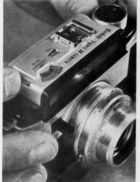
**EXPOSURE METER** was designed to be integrally mounted on a new Kodak camera.
