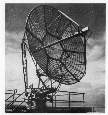
**TROPOSPHERIC SCATTERING**, given special attention in a study of the propagation of radio waves, is traced by an antenna at the Research Laboratory, Schenectady.
