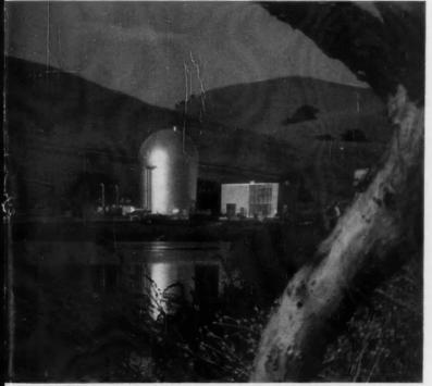
Vallecitos Atomic Laboratory boiling-water reactor powers 5000-kw turbine-generator.
