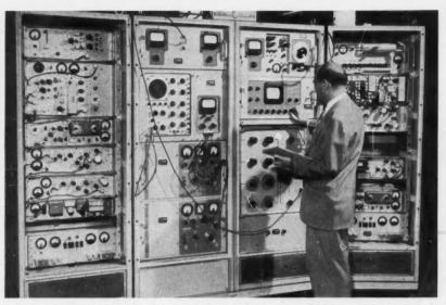
**RACKS OF EQUIPMENT**, developed with Lincoln Laboratory of MIT for U.S. Air Force's new tropospheric scatter UHF communications system, have a 700-mile range.
