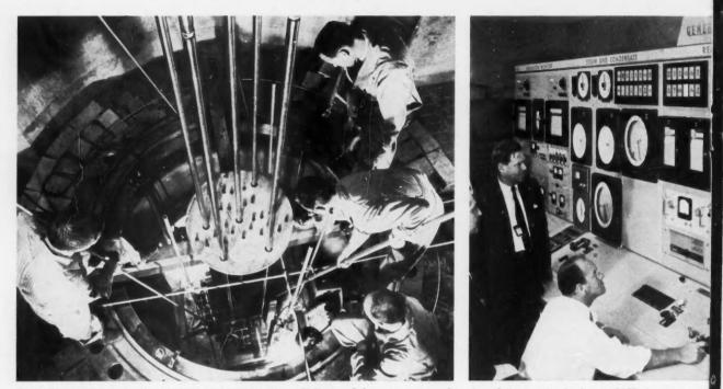
DEVELOPMENTAL BOILING-WATER POWER REACTOR at Vallecitos Laboratory sustained its first chain reaction in August 1957; instruments
