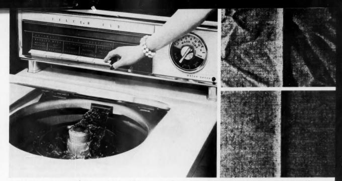
**AUTOMATICITY IN APPLIANCES** increased during 1957. A new automatic clothes washer was equipped with 5 push buttons to produce a combination of variables covering any conceivable clothes load.
