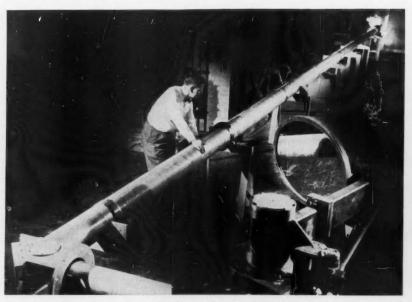
PERISCOPE, believed to be the world's longest, has a 90-foot aluminum tube equipped with intricate mirror-and-lens system for safe viewing of a reactor undergoing test.
