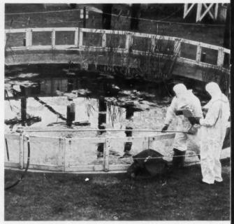
**PLASTIC SHEATH** seals off radioactive equipment when removed from waste storage tanks, prevents spread of radioactive contamination.
