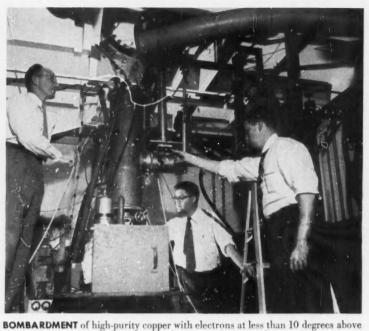
absolute zero provides improved test of radiation damage at low temperatures.
