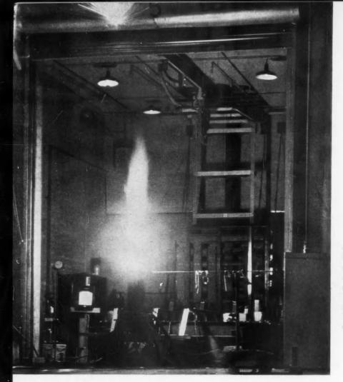
Newest stabilized plasma jet, believed largest in free world, blasts gas plasma at 26,000 F at larger re-entry vehicle models in improved simulation of flight between Mach 12 and 25. Four times larger than previous units, the jet consumes 15,000 kw—enough alternating current for 5.4 million homes.
