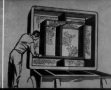
NEW ACOUSTIC TREATMENT for large high speed motors reduces high-frequency "whine" to a quiet hum, improving employee comfort, efficiency. GEA-6571.
