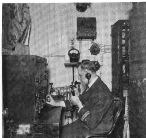
Fig. 4. Another View of the Installation on Board the S. S. America
