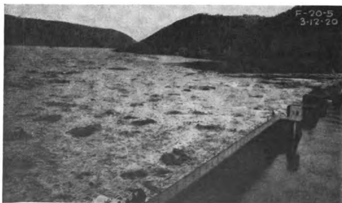
Fig. 4. Cake Ice Does Not Ordinarily Affect Hydro Plant Operation. This illustration shows how an arched wall prevents the ice from getting into the forebay
