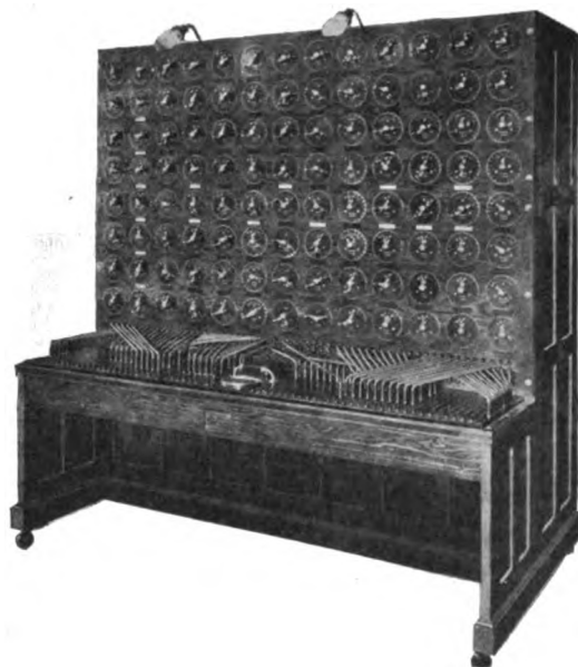
Fig. 21. Short Circuit Calculating Table
