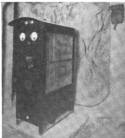
Fig. 5. "Safety First" Charging Panel in a Copper Mine
