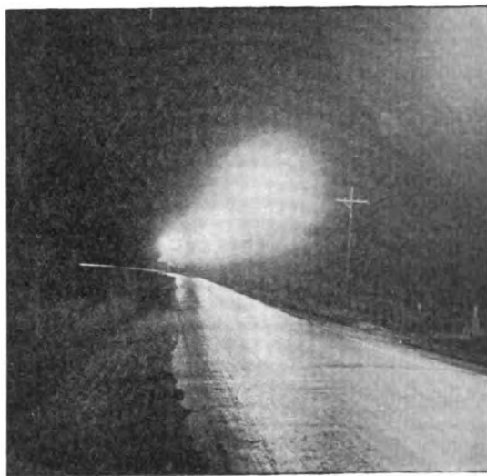
Fig. 7. Night View of Paradise Road, Swampscott, Mass., Illuminated by Novalux Highway Units Equipped with 2500-Lumen (250-c-p.) 6.6-amp. Mazda C Series Lamps
