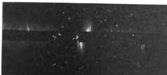
Fig. 19. Corona at 900-kv. 3.5-in. (8.9 cm.) Diameter Tube 144-in. (366 cm.) Spacing
