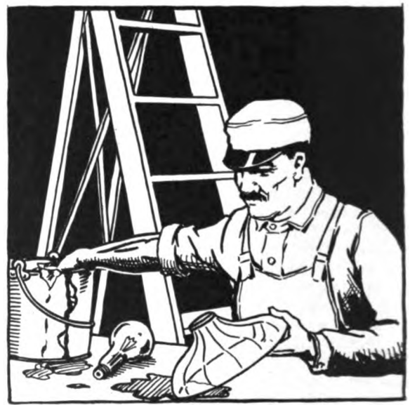
Fig. 6. Equipment should be thoroughly cleaned at regular intervals, the frequency depending upon the location
