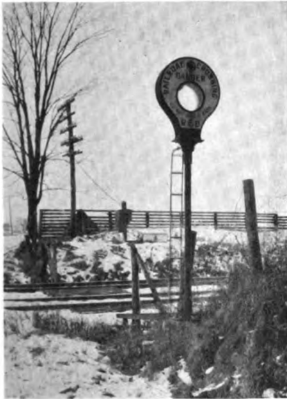
Fig. 78. Relay Operated Flashing Danger Signal at Railway Crossing
