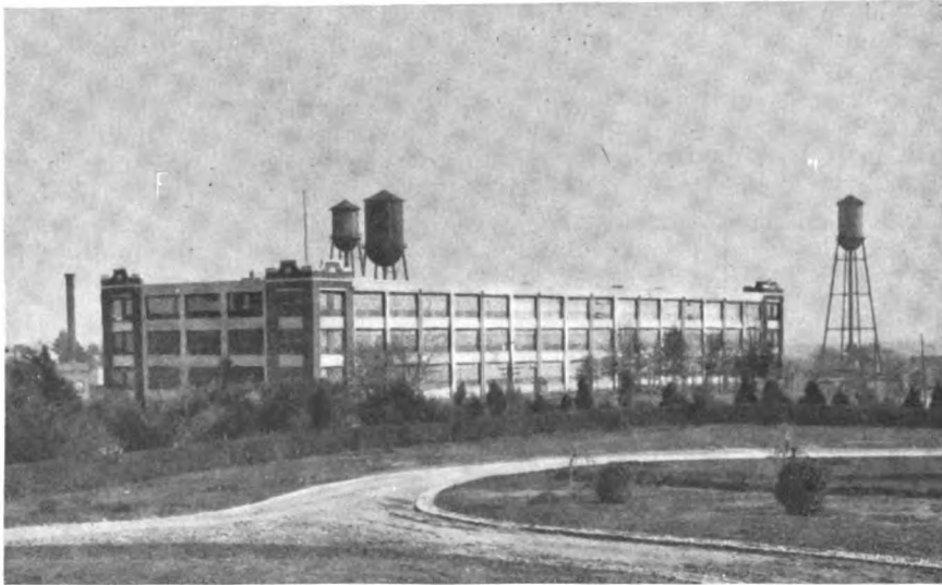
Fig. 1. Modern Cotton Mill Building. This mill, equipped with individual motor drives in picking, spinning and weaving departments, has been in operation since 1917
