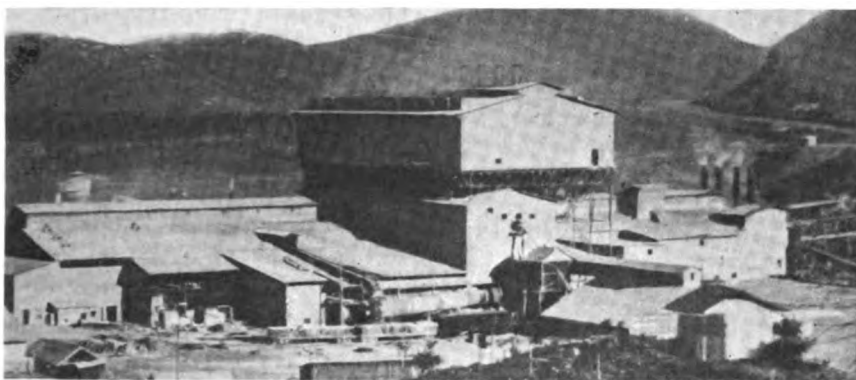
Fig. 3. Photograph of the Riverside Portland Cement Company's Plant Taken After Cottrell Precipitator Equipment was Installed
