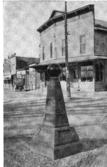
Fig. 79. Battery Operated Highway Guide Post
