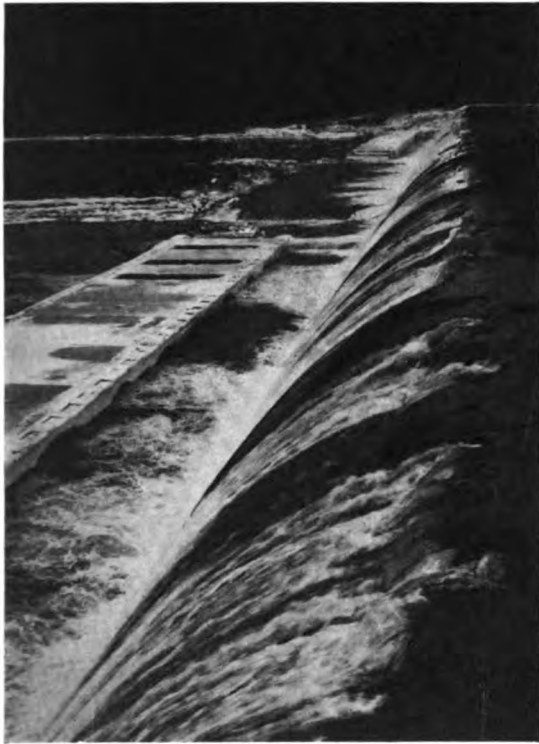
Fig. 5. Anchor Ice Adhering to the Crest of a Dam
