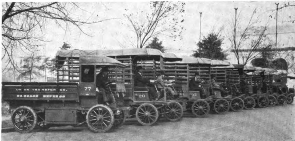
Fig. 6. Baggage Express and Transfer Trucks (Commercial Truck Company)
