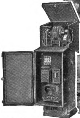
5- to 70-kv-a., 2300-volt; Automatic Regulator for Outdoor Installation
