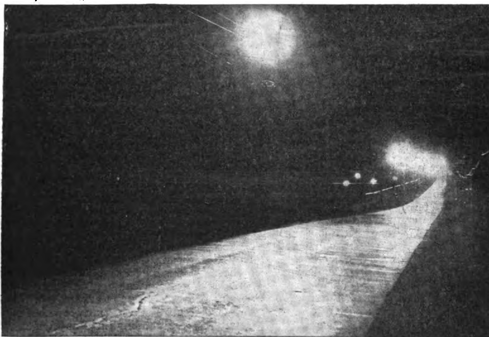
Fig. 82. A Typical Installation of Highway Lighting Units
