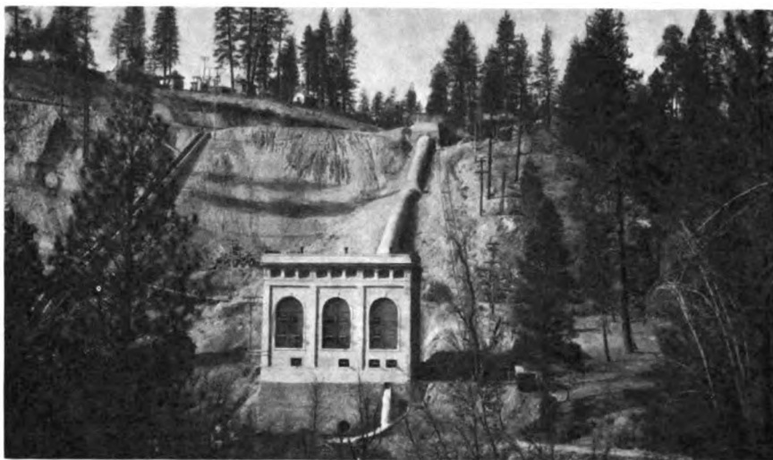
Fig. 1. Hat Creek Power Plant No. 2, Pacific Gas and Electric Company. This is a Stream Flow Plant, there being no dams or reservoirs in connection with the water supply. Installed capacity 12,500 kv-a.
