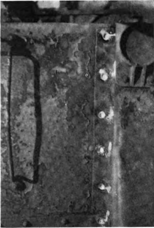
Fig. 2. Rivet Heads burned flush with surface of car
