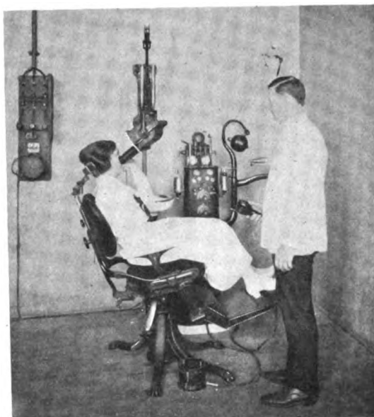
Fig. 40. Dental Oil Immersed X-ray Outfit in Use
