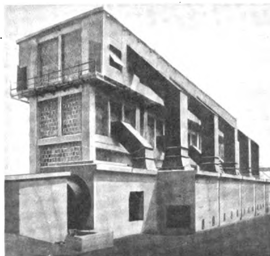
Fig. 1. Cottrell Precipitator Installation for Treating Cement Kiln Gas at the Dexter Portland Cement Company, Nazareth, Pa.
