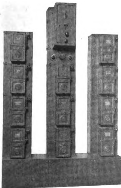
Fig. 64. Switchboard Built Up of Safety Enclosed Lever Switches
