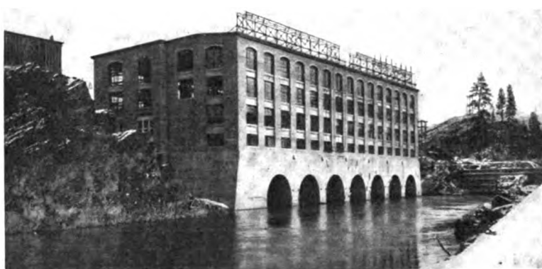
Fig. 6. Thompson Falls Power House and Tailrace of Thompson Falls Power Company, 30,000 kw., 55-ft. head
