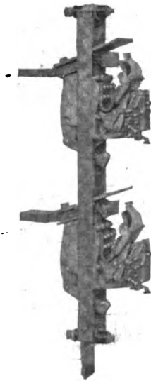
Fig. 52. 2400-amp., 250-volt Direct-current Circuit Breakers Mounted on Feeder Bars
