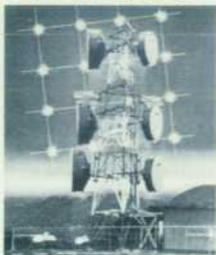
Behind many of the microwave antenna towers one can see riding the tops of ridges and tall buildings are digital radio systems, that is, systems in which the information is imposed on the microwave carrier signal by digital modulation techniques. Two instruments for testing digital radios are the subjects of this issue.
