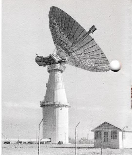
*Fig. 4. Ballistic missile early warning radar at the Lincoln Laboratory of M.I.T. Using the klystron shown in Figure 5, this installation made radar contact with planet Venus.*
