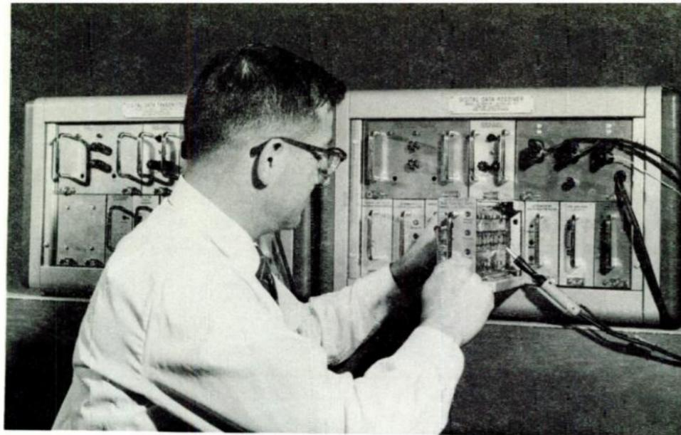
*Figure 4. Commercial prototype of high speed data transmission terminals. This equipment has transmitted data at 3360 bits-per-second rate within a single carrier voice channel having a useful bandwidth of less than 3000 cycles. Path length was 450 miles. No errors occurred in transmissions exceeding ten million bits.*
