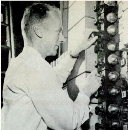
*Figure 1. Antiques of communication, these 22-A-1 voice frequency repeaters were put in service 37 years ago, one year before Chief Transmission Man D. L. Hensley, shown inspecting, was born. This long service typifies telephone industry insistence on reliability and compatibility between old and new. Electron tubes shown are relatively new, having been substituted for an older version about 1929. Repeaters still worked perfectly when retired from service recently.*
