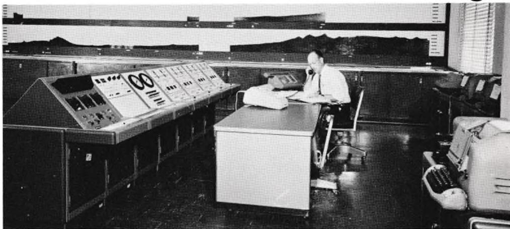
*Figure 5. A typical centralized control station for a pipeline. From this location are monitored such operational details as flow rate, pump pressure and suction, fluid viscosity, and the like. Distant operations can be adjusted in response to changing loads and other variables. Panels in background show profile of terrain which pipeline traverses, and which has important bearing on operating parameters. Centralization is made possible by efficient digital transmission.*
