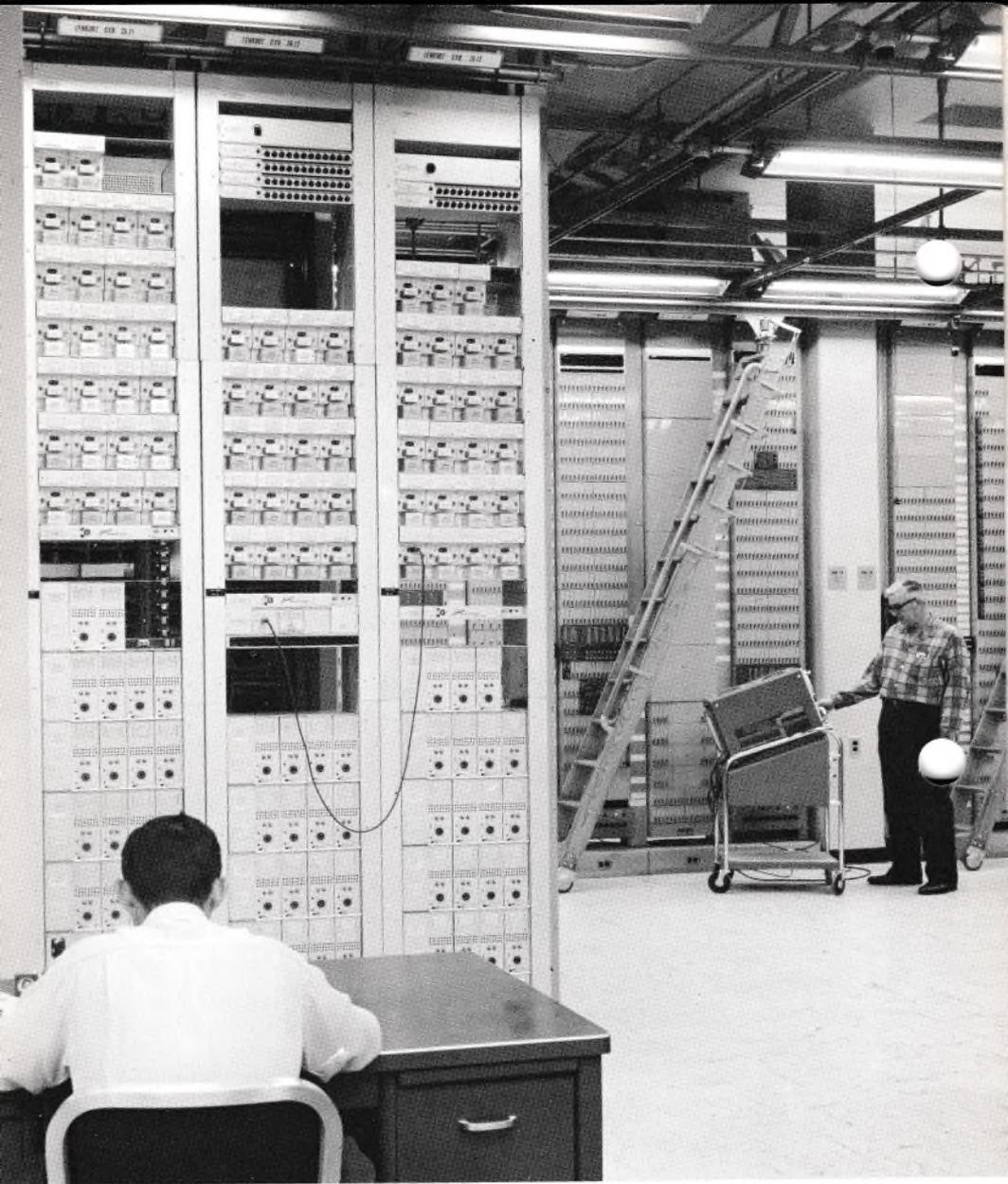
*Figure 6. California end of Hawaii-mainland submarine cable. In background are some of the racks for TASI system which squeezes waste time out of conversations to obtain additional voice circuits from the limited cable bandwidth. In left foreground is the Lenkurt 23A Telegraph Carrier system which provides signaling and supervision for the TASI voice circuits. The 120-cycle channel filters permit 22 to 26 signaling channels or 100-speed telegraph channels to be sent through each voice channel.*
