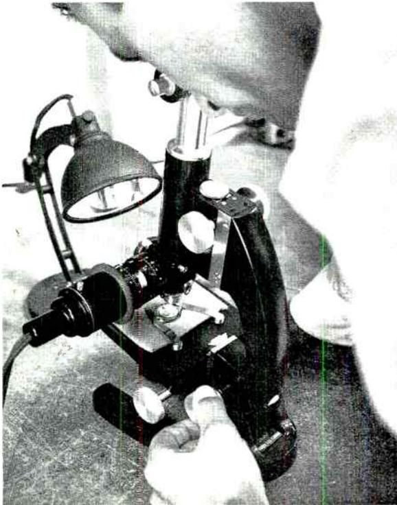
*Figure 5. Transistors that fail during operation are examined and tested in Lenkurt's Material Evaluation Laboratory. If electrical tests do not reveal the cause and mode of failure, the transistor is cut open, potted, and then slowly abraded and polished until the physical defect can be seen under a microscope. Cause of failure can usually be determined by viewing the damaged area of the transistor.*
