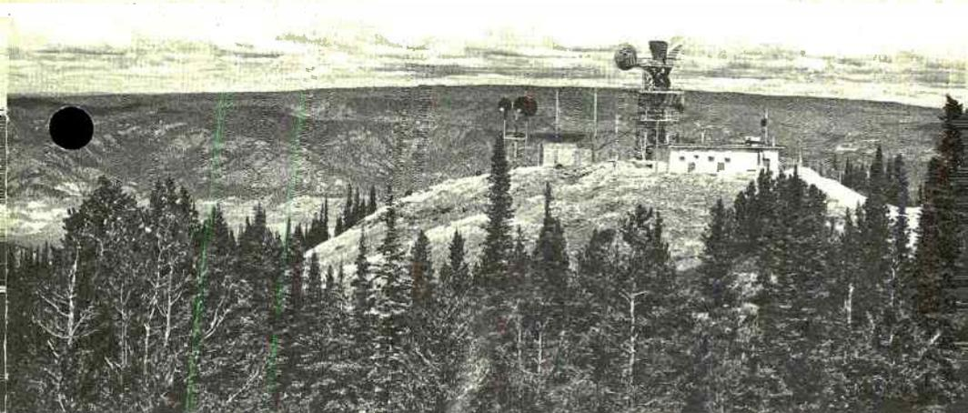
*Figure 5. Often, microwave radio stations are located in isolated areas where public or commercial power is not available.*
