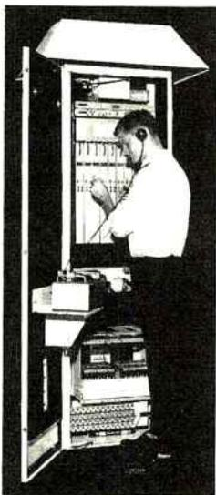
Lenkurt's 565 weatherproof cabinets offer complete protection of telecommunication equipment in all outdoor installations. Temperature and moisture control, insulation, and rugged construction make the 565 cabinet a comfortable home for your equipment in any climate, on pole or pedestal.
