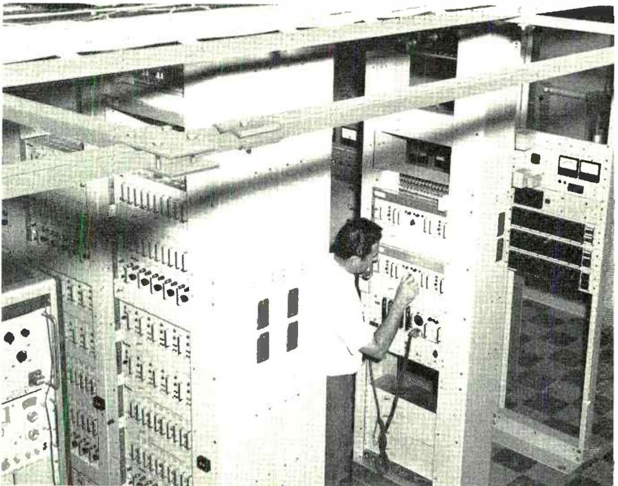
*Figure 7. Row upon row of communications equipment fills key stations in the instrumentation and data control system. Here, technician checks Lenkurt multiplex and signaling equipment at White Sands.*
