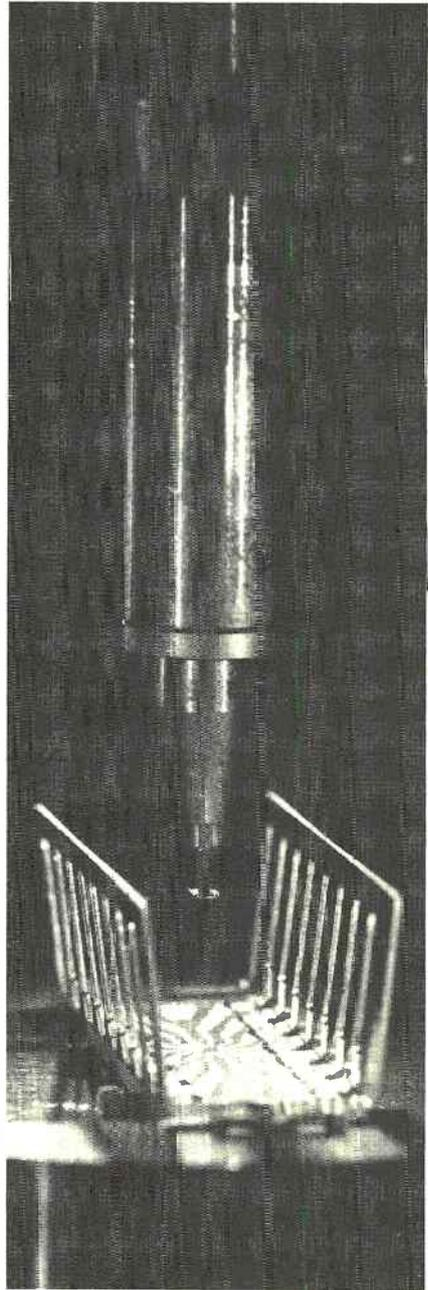
*Figure 6. Recently developed technique shows Fairchild integrated circuit about to be mounted face down on frame. All contacts are made at one time.*
