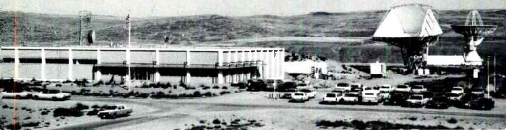
*Figure 1. Brewster Flat ground station, with folded-horn and Cassagrain antenna (right, in distance). Microwave antennas are visible above building.*
