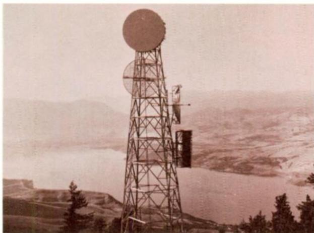
*Figure 2. Microwave repeaters operate unattended from the tops of mountains.*
