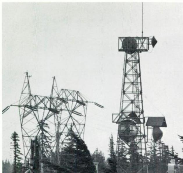
*Figure 6. Electric utilities use microwave systems to monitor current flow along transmission lines.*
