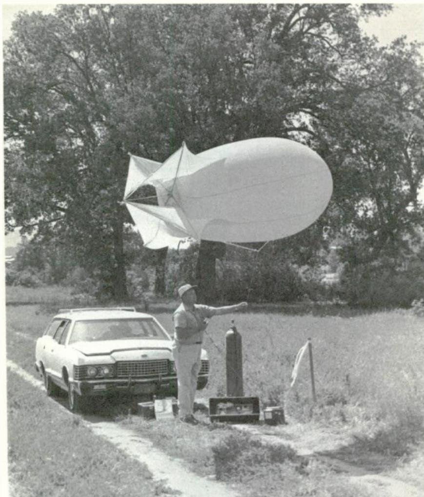
*Figure 4. The auxiliary equipment needed for “balloon” flying includes a helium source, VHF radio, and a calibrated, motor-driven reeling mechanism.*
