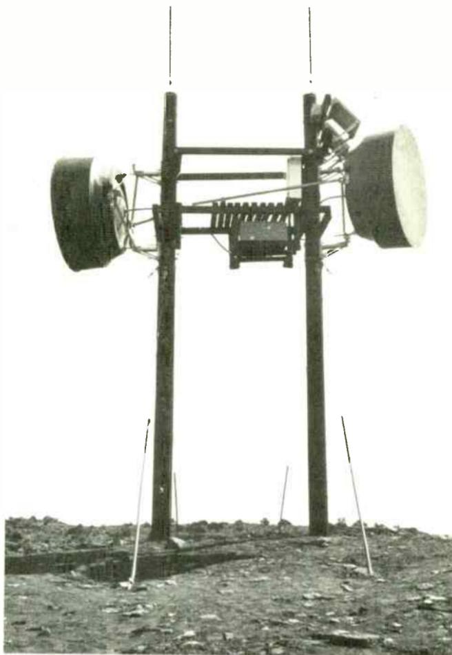
Expensive housing is unnecessary for the 700F1, which operates over a temperature range of  $-40^{\circ}\text{F}$  to  $+140^{\circ}\text{F}$  and has all its active components mounted in a weatherproof metal box. Since the 700F1 uses a minimum of components, it is more reliable than conventional repeaters; in addition, the entire system is 100 percent actively redundant.
