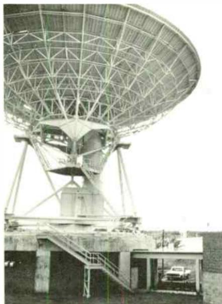
Figure 2. Antenna with track and wheel assembly – Palamu, Hawaii Earth Station.
