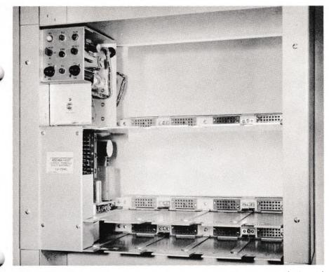
FIG. 4. Type 45CB terminal shelf with plug-in units removed. The Power Distribution and System Alarm Unit is permanently wired to a short section of cabling which permits its partial removal from the shelf for inspection and maintenance.
