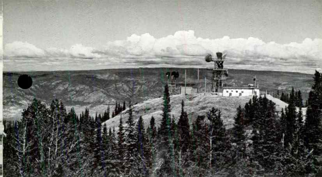
Figure 5. Often, microwave radio stations are located in isolated areas where public or commercial power is not available.
