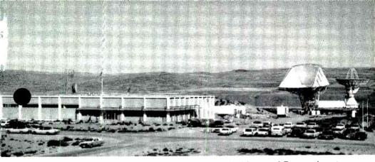
Figure 1. Brewster Flat ground station, with folded-horn and Cassagrain antenna (right, in distance). Microwave antennas are visible above building.
