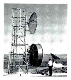
The Pacific portion of the Comsat global communications system is being linked to major telephone switching networks with Lenkurt microwave radio.
