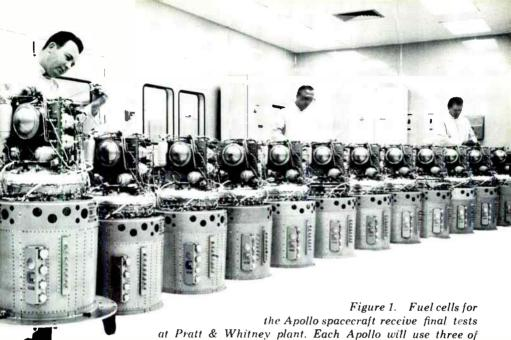
these units, producing up to 2 kW each from pure hydrogen and oxygen.
