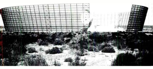
Figure 1. Radar is first range instrument to "see" missile. Installation at White Sands Missile Range is surrounded by clutter shield.
