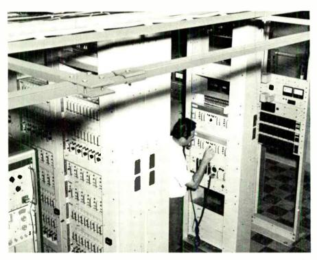
Figure 7. Row upon row of communications equipment fills key stations in the instrumentation and data control system. Here, technician checks Lenkurt multiplex and signaling equipment at White Sands.
