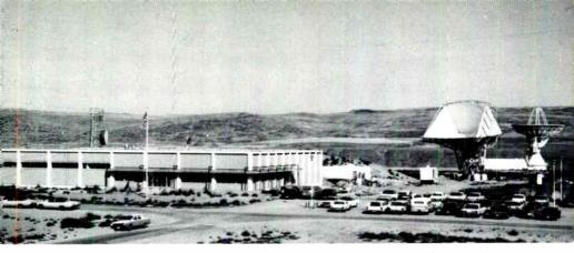
Figure 1. Brewster Flat ground station, with folded-horn and Cassagrain antenna (right, in distance). Microwave antennas are visible above building.
