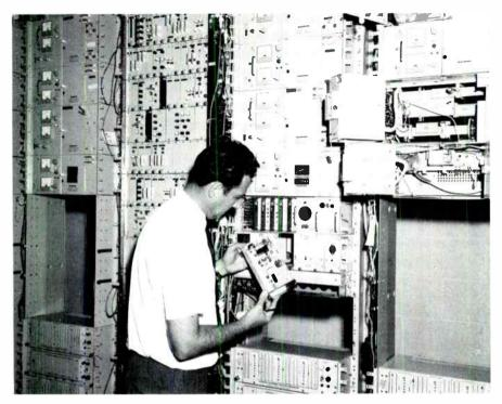
Figure 5. Lenkurt 76 microwave radio system provides updated communications capabilities at White Sands Missile Range. To left of radio is 57B path protection system.
