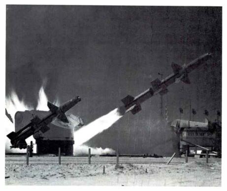
Figure 6. Short and long range missiles must undergo the same demanding tests before they become operational. Here, the TALOS is fired from a simulated ship at White Sands. The missile is under constant surveillance as it passes over the range.
