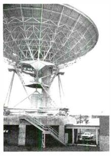
Figure 2. Antenna with track and wheel assembly — Pamalu, Hawaii Earth Station.
