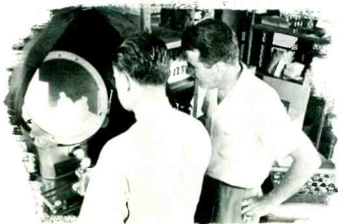
An optical comparator is used to inspect the machined head of an x-ray tube cathode. This instrument not only shows an enormously magnified silhouette of a small metal part, but by means of a projected scale enables the operator to measure the part with ten-thousandth-of-an-inch accuracy.
