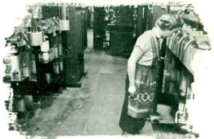
Believe it or not, this is a foundry! The personable young lady in the dainty apron is overseeing the high-vacuum induction casting of copper anodes—a process developed by Machlett Laboratories and unique to Machlett Laboratories.
