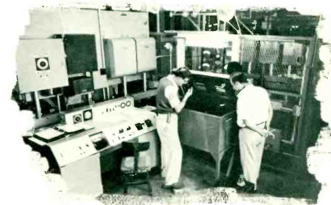
X-ray tubes are tested under high voltage in an oil-immersion tank.
