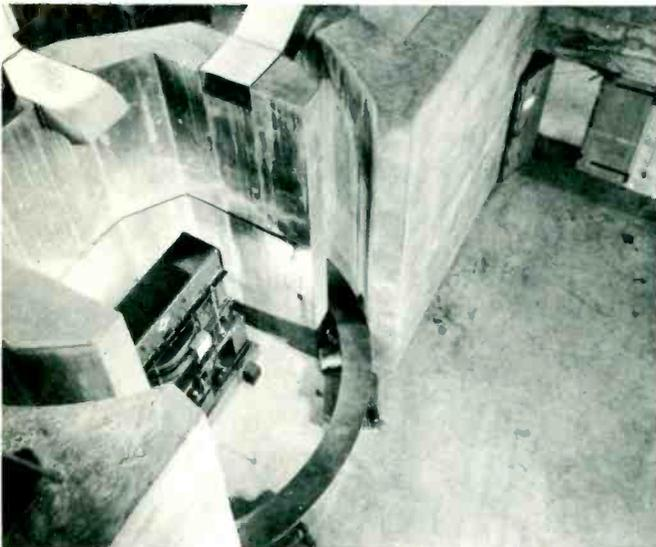
A Betatron in position, surrounded by great shielding walls of concrete to guard against uncontrolled radiation. The Donut is between the two curved-edge parts at left center of the apparatus.
