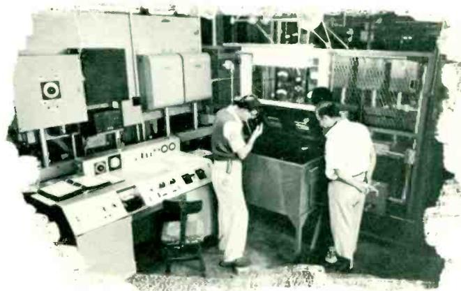
X-ray tubes are tested under high voltage in an oil-immersion tank.
