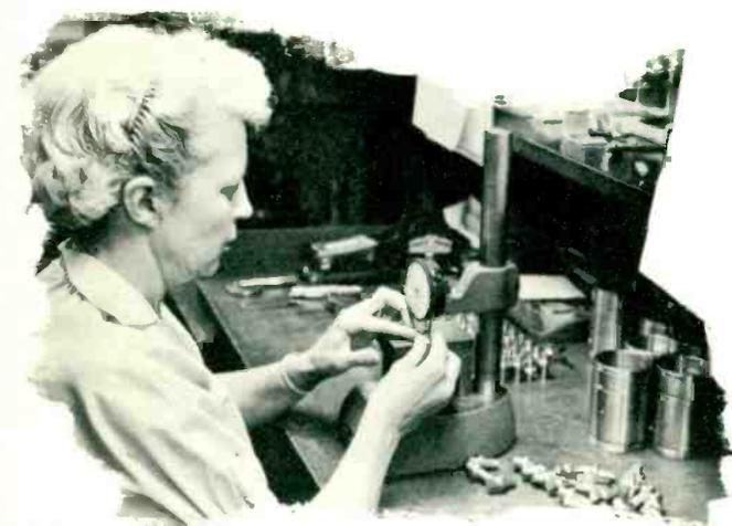
Purchased parts are inspected on receipt and tested with micrometers and other precision measuring equipment before being put into stock.
