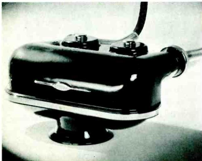
Early Dynamax model which appeared on the market in 1939 and was to prove the most efficient tube for general radiographic applications.
