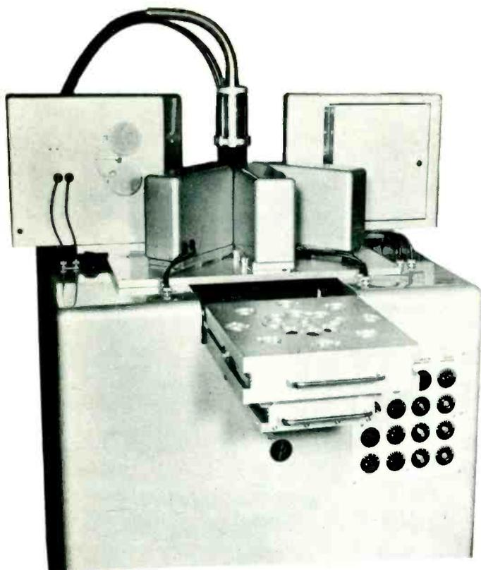
Applied Research Laboratories' x-ray spectrometer utilizing Machlett beryllium window tube.
