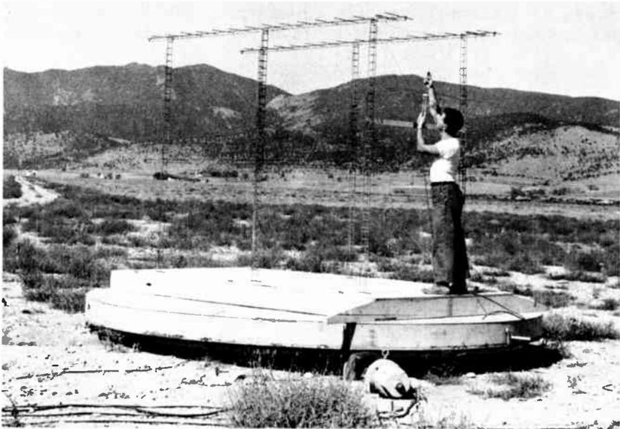
*Figure 4. Scale Model of Huge Yagi Array Shown in Figure 3*
