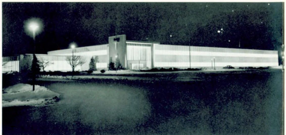
Computer Division, Willow Grove, Pa. Building completed and occupied February, 1960
