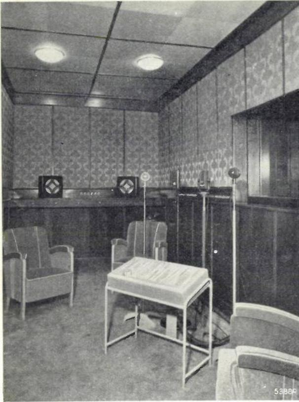
Fig. 4. Microphone room (C in fig. 2), with four different types of microphones. In the foreground a movable switch panel with push-buttons and pilot lamps. The two loudspeakers (in background) have been designed for radio relay.
