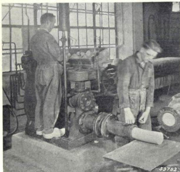
Fig. 2. De-airing pug-mill in operation.
