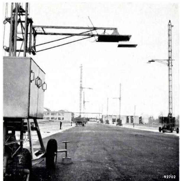
Fig. 1. Daylight view of the Philips open-air laboratory for road lighting.
