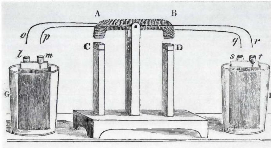
Fig. 6. Henry's reciprocating electric engine (1831). The reciprocating electromagnet *AB* is alternately connected to the batteries *F* and *G*. Attraction and repulsion between the electromagnet and the permanent magnets *C* and *D* maintain a continuous motion.
