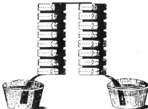
**Fig. 1.** The voltaic pile, as illustrated in the first publication (in *Phil. Trans. R. Soc.* 90, 403, 1800)<sup>[1]</sup>. A stands for silver (argent) and Z for zinc.
