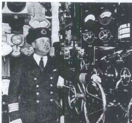
Chief Engineer Melroy at Control Switchboard of Queen of Bermuda
