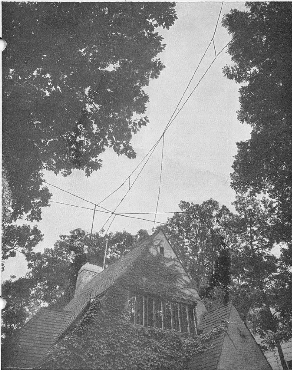
View Showing the Two Antennas, One Facing E. and W., the Other Facing N. and S.
