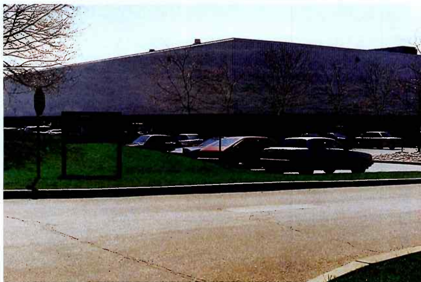
Fig 1: Nulogix Technical Services Inc. in Toronto is the largest depot repair company in Canada.
