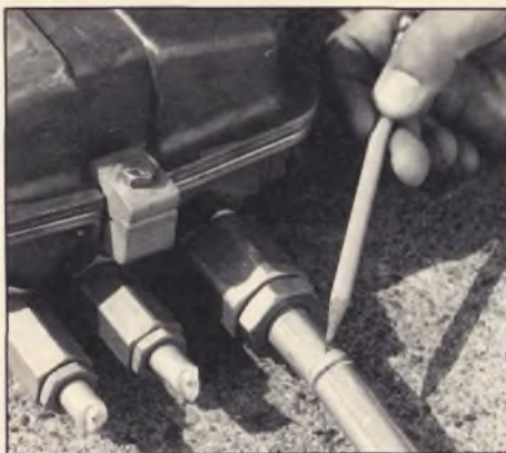
Fig. 2: The Channel 6 ingress problem was traced to a cable connection that had been stressed. In the constantly changing environment, there is no perfect cable fitting.
