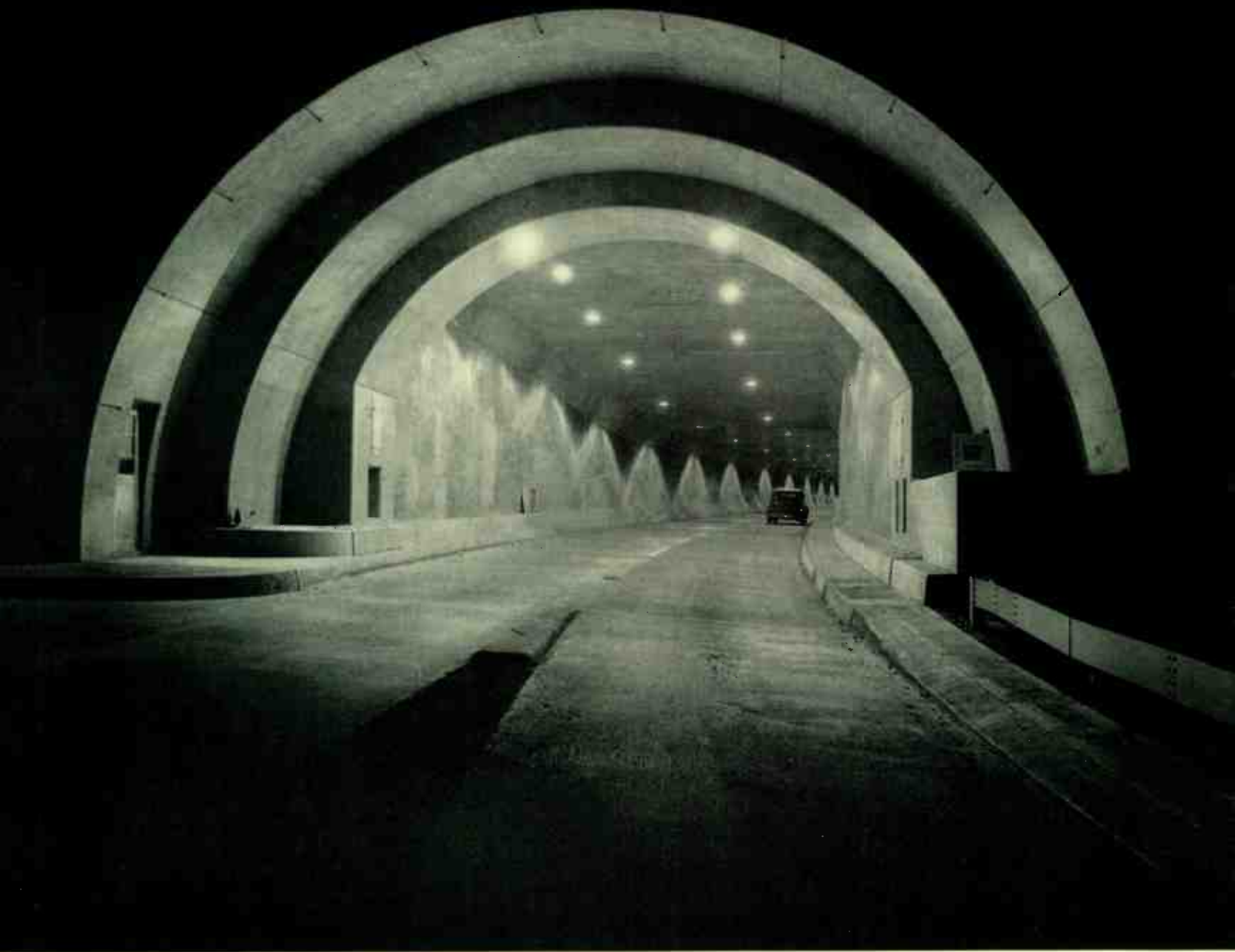
The new Harrisburg to Pittsburgh Turnpike gives a preview of the highways of tomorrow. Conspicuous among the innovations is the lighting of the tunnels and interchanges. The seven tunnels, totaling seven miles, are lighted by special 250-watt mercury-vapor lamps.
