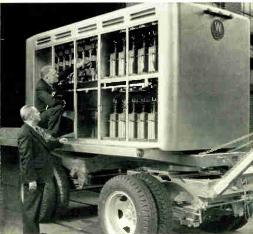
This is not a streamlined mobile circus cage for wild animals. Instead it contains capacitor units with which distribution engineers can set out on a safari for lurking low power factor. This one is for the Allentown district of the Pennsylvania Power and Light Company.
