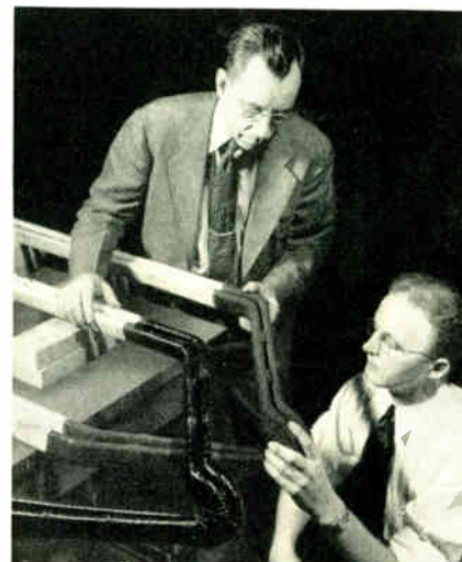
Drs. Hill and Berberich with high-voltage generator coils. The right pair has been treated to prevent the formation of corona.
